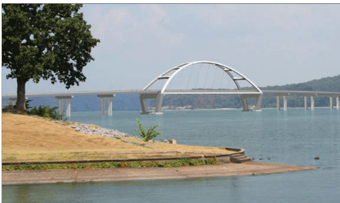
The conceptual rendering above features the unique basket-handle tied arch design that will replace the Eggners Ferry Bridge over the Kentucky Lake in the coming years. An identical bridge will couple over Lake Barkley.
